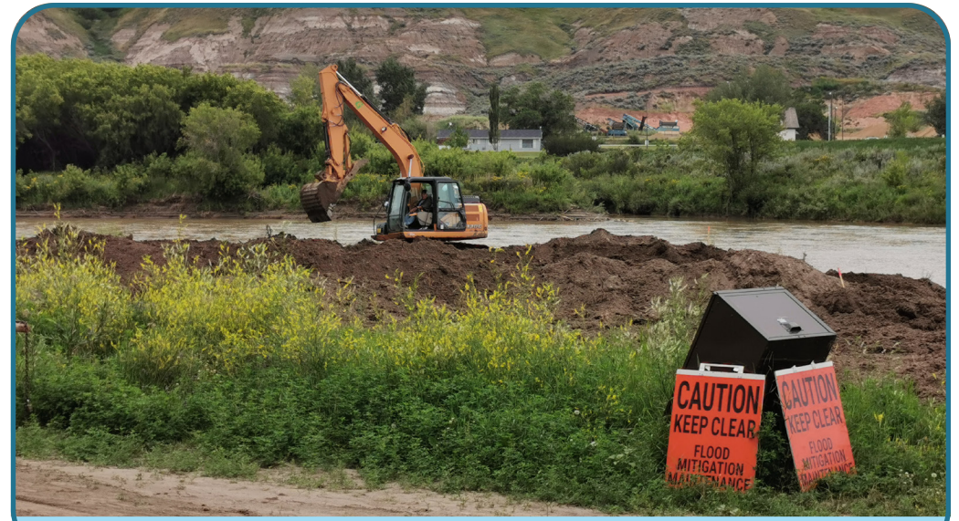
Flood mitigation work at Newcastle Recreation Area, July 2020
