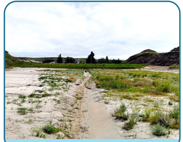
Storm Detention Pond, August 2020
