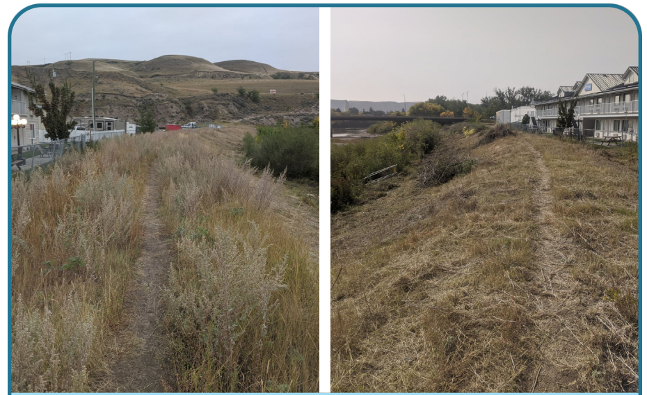
Dike C brush clearing: before (left) and after (right), September 2020
