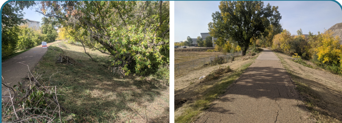
Dike D brush clearing: before (left) and after (right), September 2020
