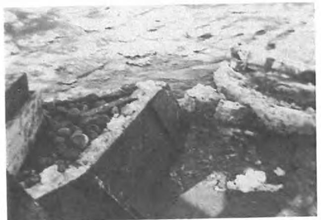
April 21, 1948, this wooden pier of the third span of the East Coulee C.P.R. bridge is starting to lose its metal plate protection from the damaging effects of the ice floes. The side metal plate is already gone, only the "V" shaped point is left remaining. Note: The piers were originally constructed of wooden pilings with a wooden framework around them. The centre area was filled with rocks as can be seen.
