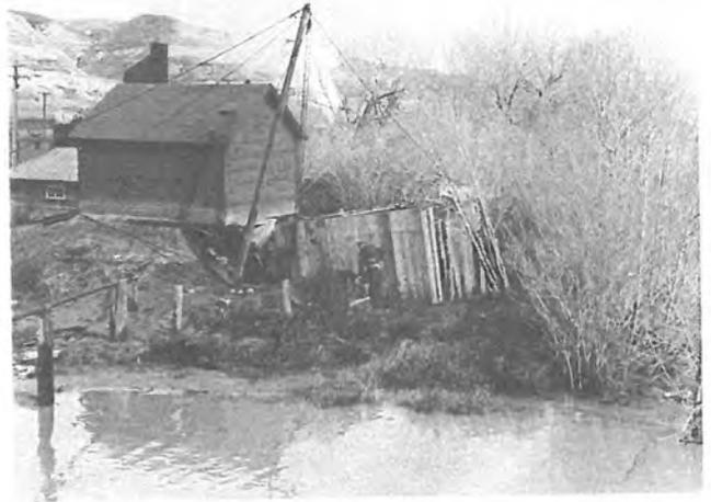
April 21, 1948, the C.P.R. pump house at East Coulee is undermined by the flood waters and ready to topple over.
