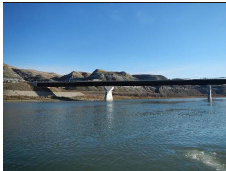
Photo 5: View downstream from Transect 6 showing the Highway 10 bridge on the Red Deer River. 31 October 2020.
