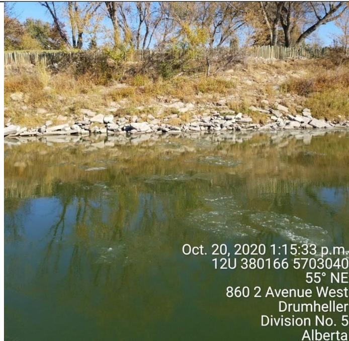
Plate 6. View of erosion along the left bank of the Red Deer River and attempts of slope stabilization.
