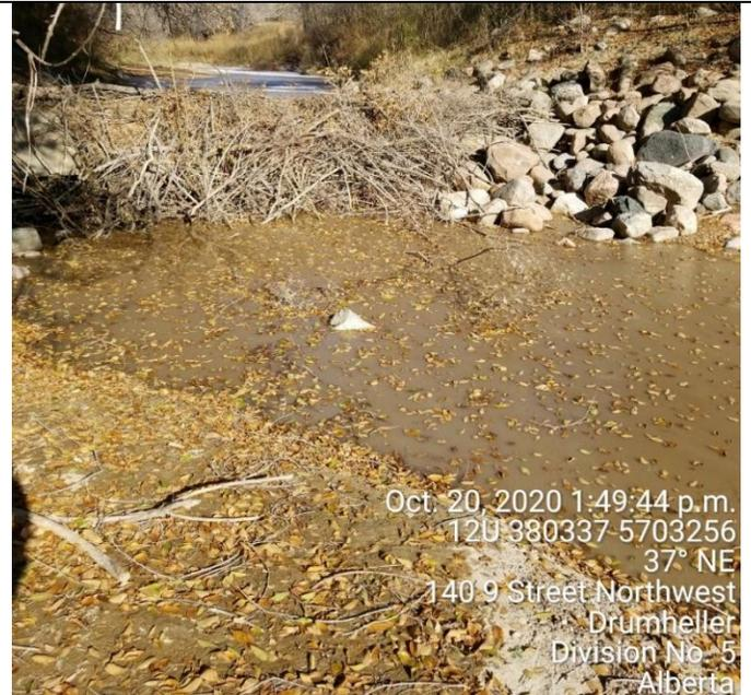
Plate 12. View of fish barrier (weir and beaver dam) at the upstream extent of the Michichi Creek mitigation footprint.
