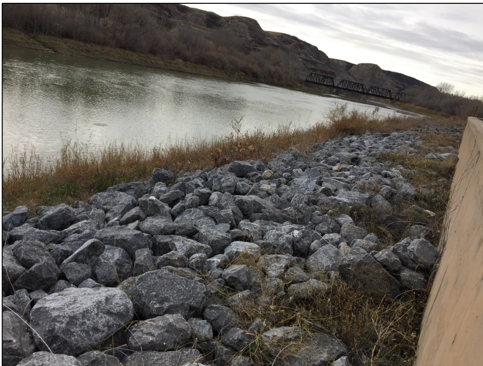
Photo 6 Armoured bank by flood control barrier present along Midland reach.
