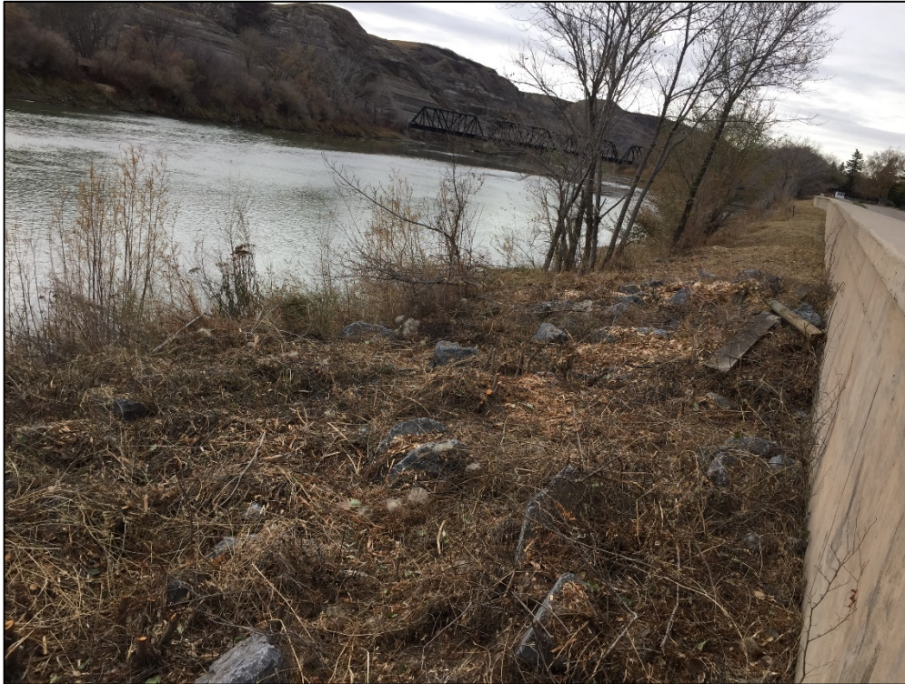
Photo 6 Armoured bank by flood control barrier present along Midland reach.
