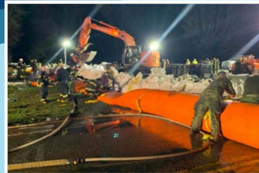
Military personnel help with the placement of a Tiger Dam on Sunday night (Nov. 28) across Highway 1 near Cole Road in Abbotsford. (PHOTO: Abbotsford Police Department)
