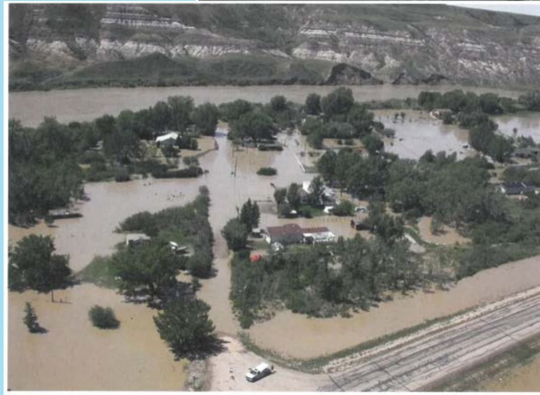
2005 Flooding in Lehigh
