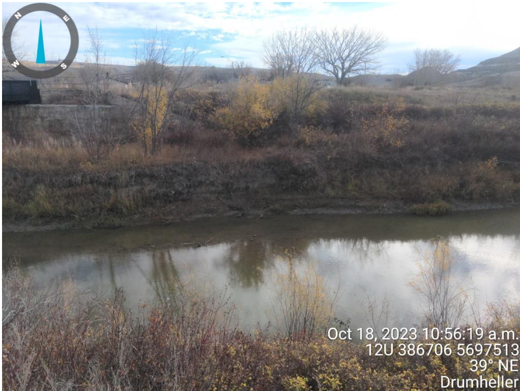
Photo 6 – View of right bank upstream of decommissioned train bridge, showing general riparian vegetation and vertical slope.
