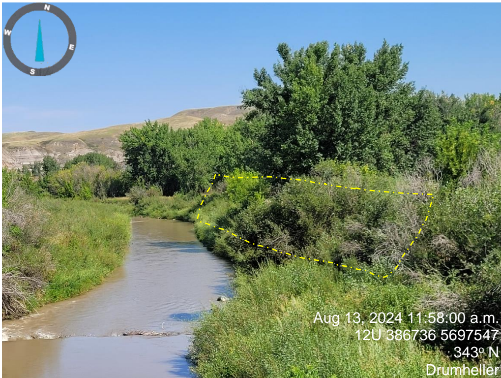
Photo 3b – Viewing downstream from train bridge at Rosedale Berm (updated August 2024).
